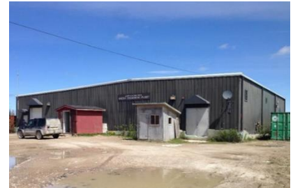
Attawapiskat water treatment plant.
