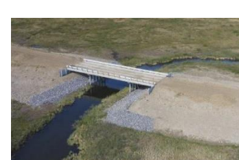
Permanent crossing over creek: Government of NWT.
