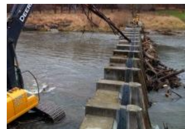
Erindale Park ice retention structure on the Lower Credit River 2
