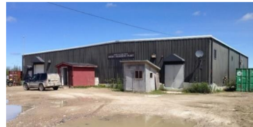
Water treatment plant in Attawapiskat.
