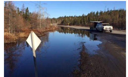
This road in Northern Ontario floods every spring, leading to closure. Photo from https://www.cbc.ca/news/canada/sudbury/hwy-537-mto-rehabilitation-1.4573211
