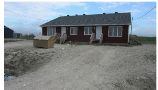
Sloping the ground around houses helps water drains away from the foundation into the ditch.
