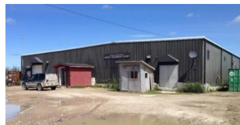
Water treatment plant in Attawapiskat.
