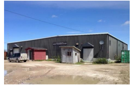
Attawapiskat water treatment plant.
